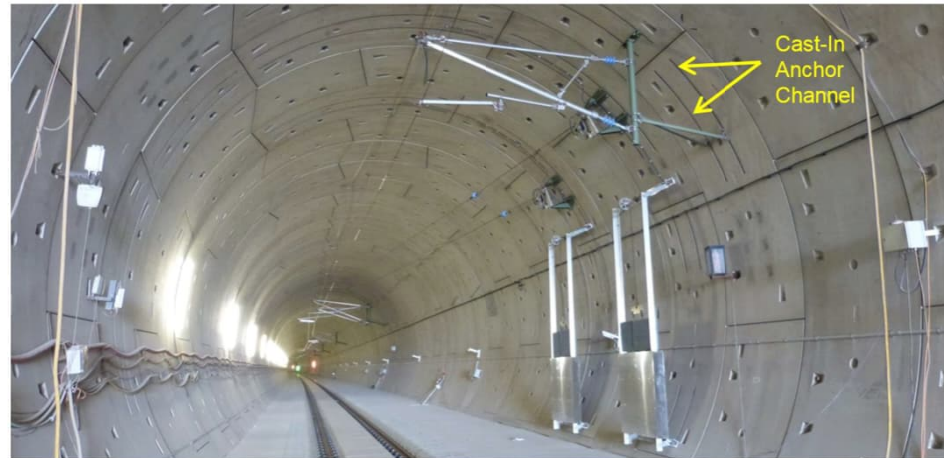
Cast-in anchors
