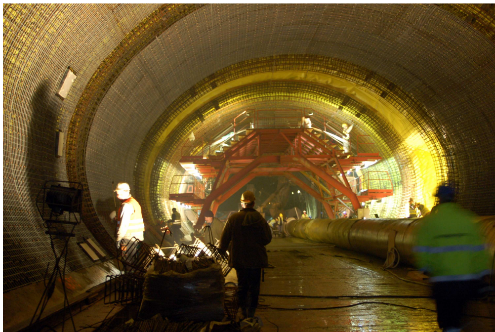
Figure 3 – The construction of Laliki Tunnel
